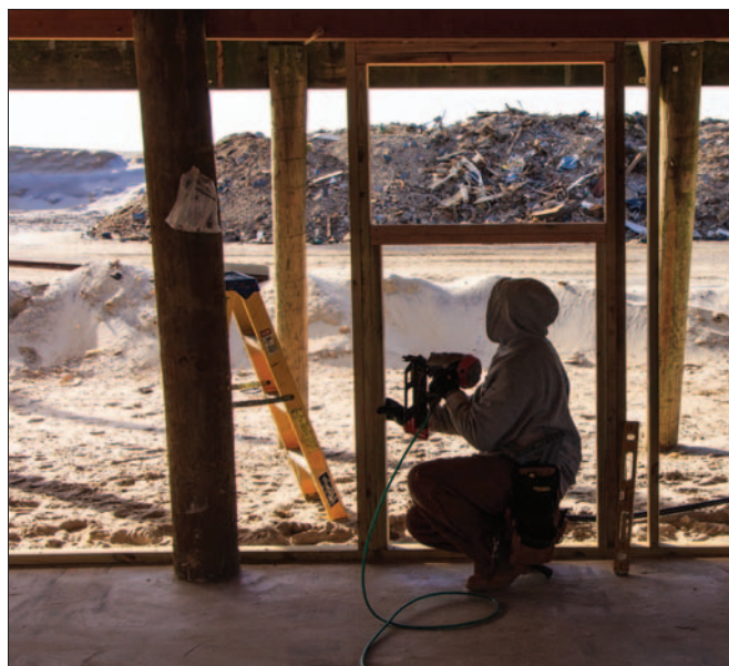
A construction worker rebuilds a home damaged by Hurricane Sandy
