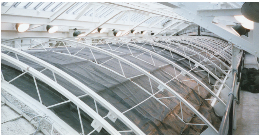
Lead-painted steel coated with Child Guard, National Gallery of Art, Washington, DC
