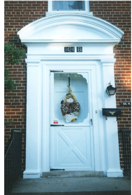
Child Guard over wood door frames at Fort Knox, KY.
