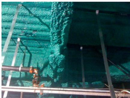
Asbestos fireproofing encapsulated to achieve abatement at the Los Angeles Federal Building. The color green was used so operations staff could readily identify surfaces to be handled with caution.
