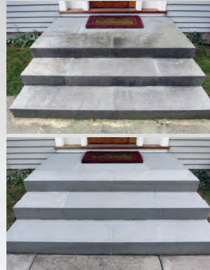
Before and after: APC with HydroBoost used to clean bluestone.
