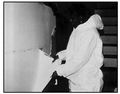
Figure 13.1 Encapsulant Failure.
