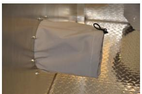
5. Bring the negative air machine inside the unit, attach it to the port flap and tighten using drawstrings.
