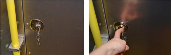
2. To exit the unit, use your thumb to push the lever to the left. The lever will unhinge from the door and open.
