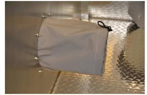
5. Bring the negative air machine inside the unit, attach it to the port flap and tighten using drawstrings.
